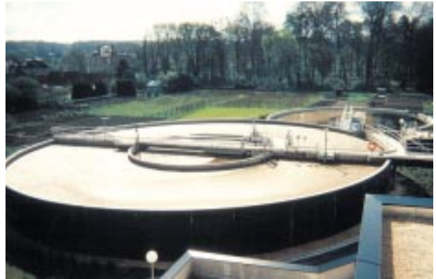
Biological phosphorus removal at Laon sewage works (North East France), Lyonnaise des Eaux. Capacity 40,000 pe.
